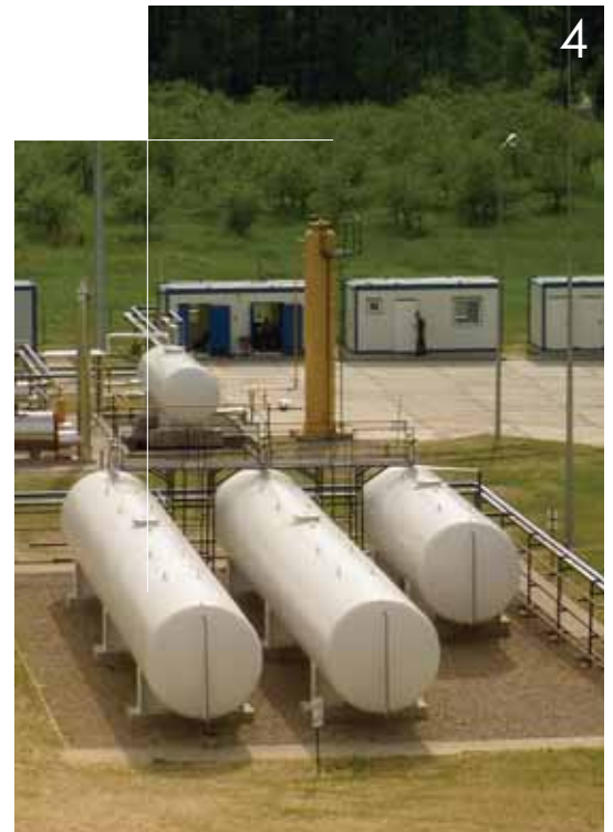
2 Crude Oil and Produced Water Storage Bullets, Gorzyca, Poland
