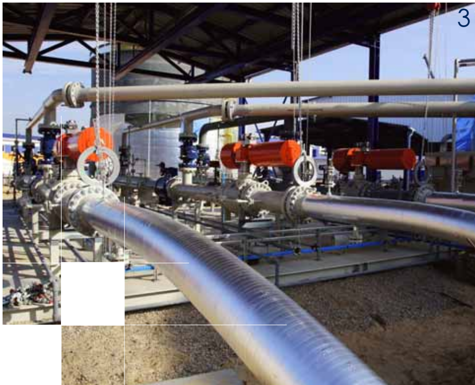
1 28" pipeline, Grodzisk, Poland 3 16/12" pig launcher, Wierzbno, Poland
