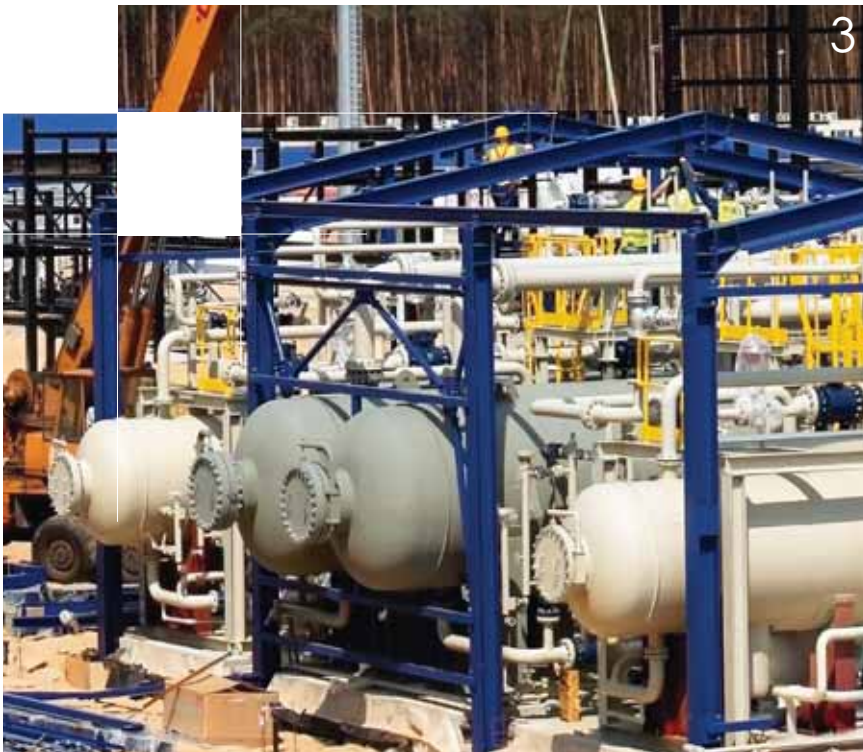
1 High Pressure Separation Unit, Miedzychod, Poland
