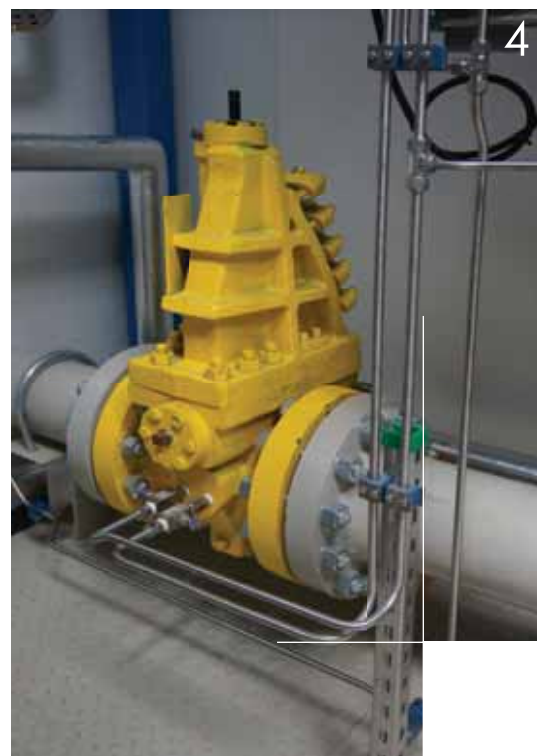
2 Ultrasonic Flow Metering Unit, Incukalns, Latvia
