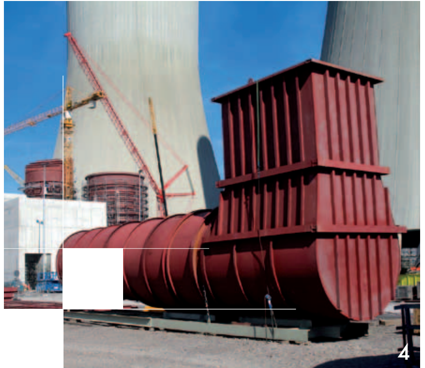
2 Assembly and installation of pressure parts at the Belchatów Power Plant, Poland 4 Prefabrication, delivery, and assembly of flue gas ducts at the Westfalen Power Plant, Germany
